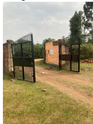
Secure Entry Gates
