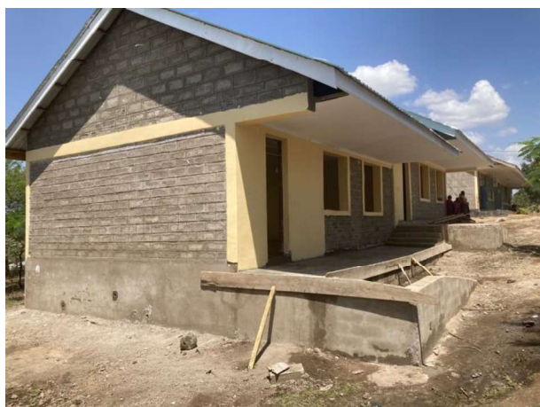
New Classrooms at Oliowang Primary School
