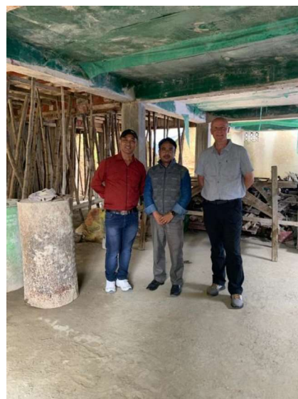
New RIBS School Facility in progress
